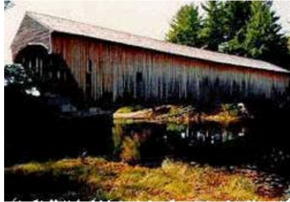
Hemlock Bridge – Maine
